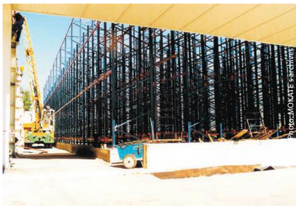
Construction of a new plant in Ustroń
