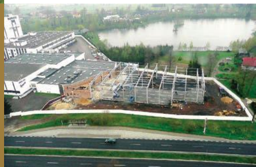
MOKATE SA in Ustroń. Production hall under construction, spring 2010
