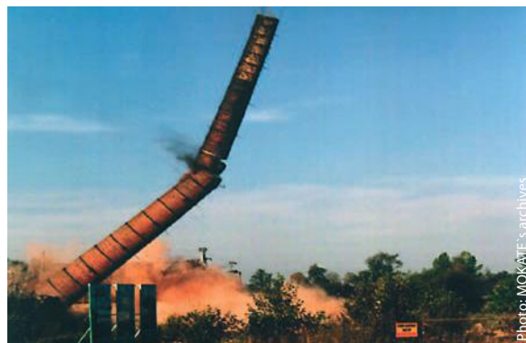
Demolition works for MOKATE's new premises in Ustron
