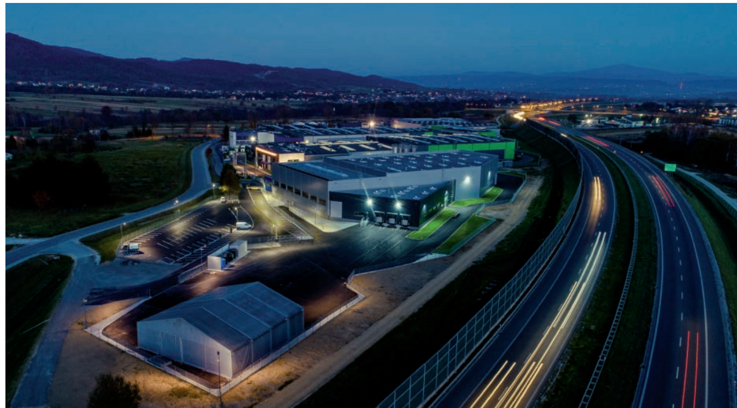
Rybarzowice – headquarter (production & warehouse)
