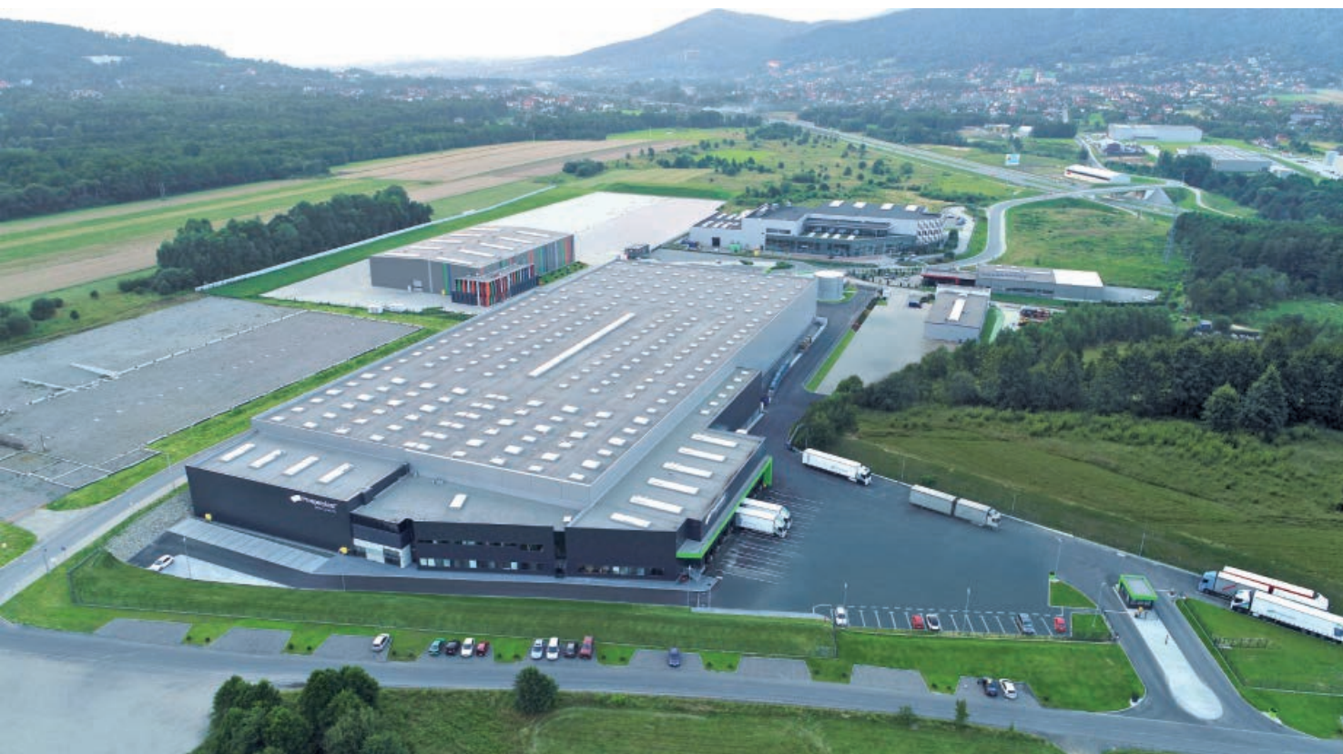
Wilkowice – logistic centre
